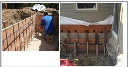
In some existing foundation situations, the structural engineer will recommend that portions of the foundation be removed and replaced with stronger foundations, or better foundation connections. This type of work is intended to gain rigidity in the foundation and lessen the impact on the structure of differential soil movement within the active zone. Underpinning and
