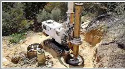
Solutions to these challenges have been designed by engineers and utilized by general contractors to permanently stabilize buildings, both large and small, new and old. These solutions include elements that attempt to connect the building to what soils engineers refer to as a “competent load-bearing strata” (referred to above as bedrock) which usually can be found below the active zone. Traditionally, to connect the
