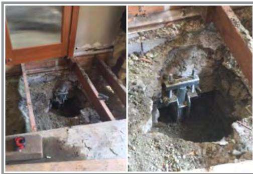
Similar foundation repair, underpinning and the use of adjustable posts *within* the footprint of a building, can be called for in areas that have settled or moved.
