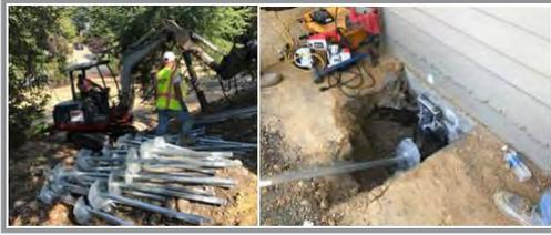
The weight of the building and the foundation itself is transferred from the unstable and expansive soils in the active zone, through the piers to the competent load-bearing strata. Moreover, the steel piers and brackets are designed in many cases to lift the foundation and thereby sometimes relevel the floors.
